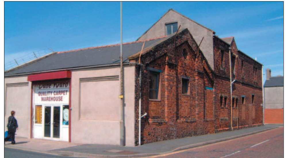
Changes to windows, in the form of uPVC windows or inappropriate designs have a detrimental impact on the proportions and balance of the elevational treatment. Changes to the size and shape of the openings themselves are even more damaging.
