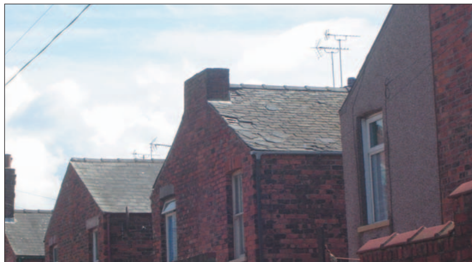
Loss of chimney stacks and pots reduces the interest of the roofline of the terraced dwellings. Lack of maintenance will also lead to water penetration and more significant damage to the property.
