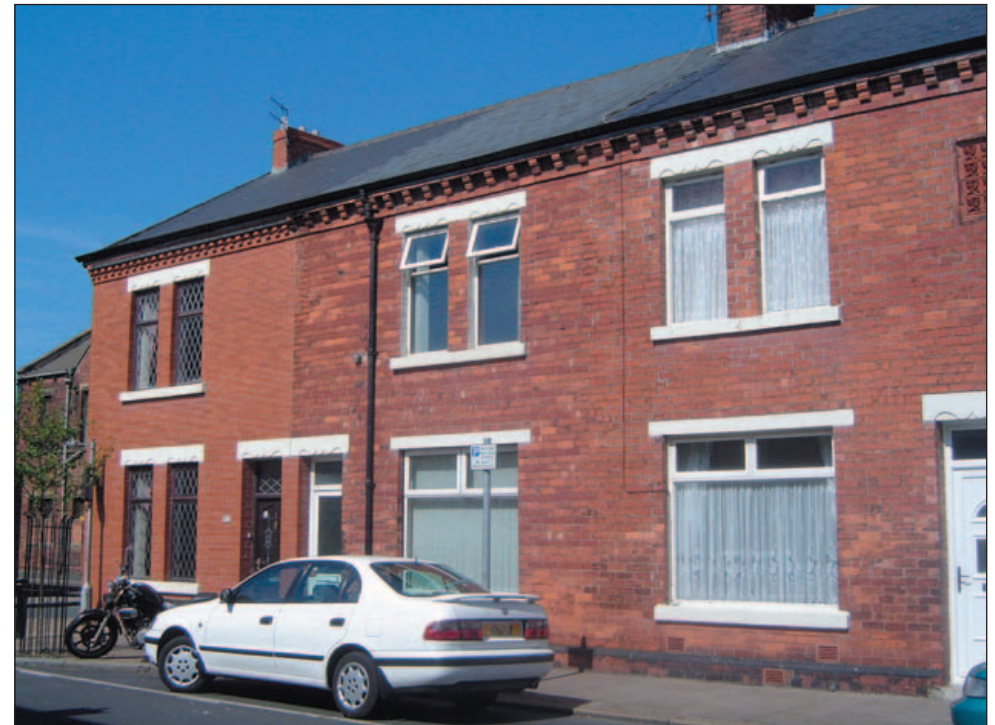
Changes to windows, in the form of uPVC windows or inappropriate designs have a detrimental impact on the proportions and balance of the elevational treatment. Changes to the size and shape of the openings themselves are even more damaging.
