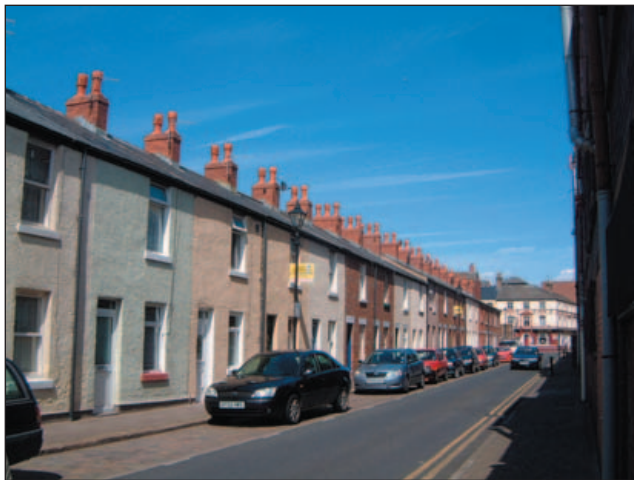
Here, the chimney stacks and pots have been repaired and/or replaced, which has a significant impact on the overall quality of the roofline. Rendered brickwork should be avoided.
